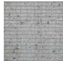
The metal lath into the concrete.
