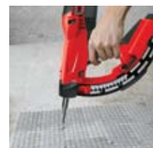
Gun in action to secure metal lath.
